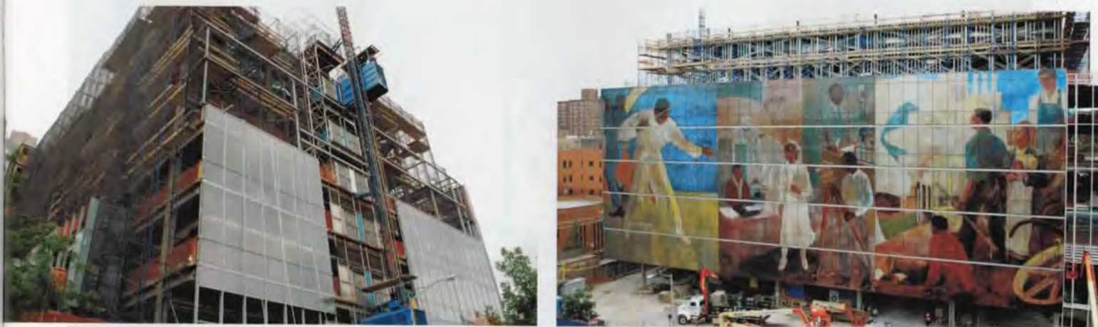
Using a new technology, the images from the historic mural were digitally printed on each 5-ft x11-ft glass panel, and the ceramic ink was then baked into the glass. The panels were laminated with a typical insulated glass unitized system, framed and then shipped to the site for installation. PHOTOS COURTESY TDX CONSTRUCTION
