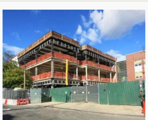
Steel structural frame construction for the new addition to P.S./I.S. 49Q., 63-60 80th Street, Middle Village – Queens, NY
